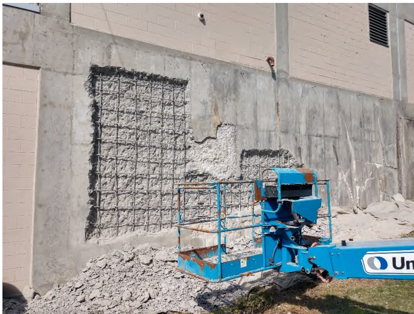
Removal of damaged exterior concrete
